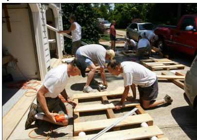
Building in the Muggs' drive.
